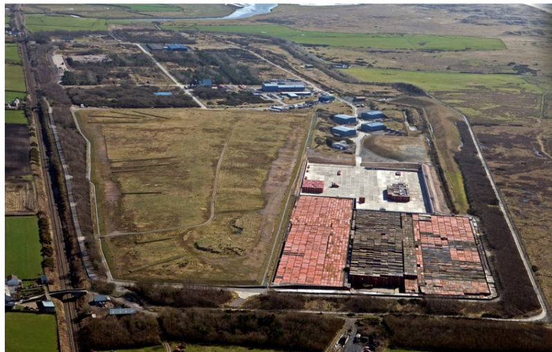
Aerial view of the LLWR showing containers in disposal vaults
