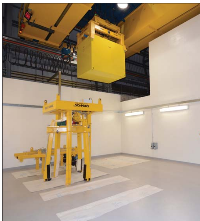
Inside the Interim Storage Facility at Bradwell
