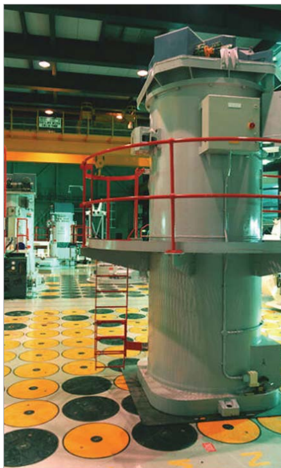
Store for packaged HLW canisters
