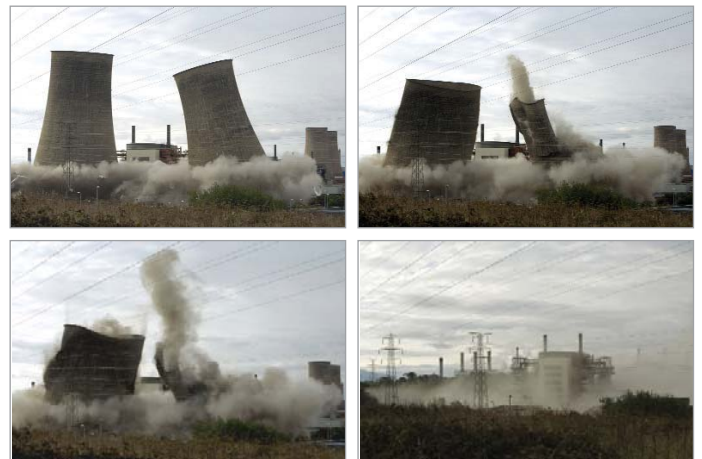
Demolition of Calder Hall towers
