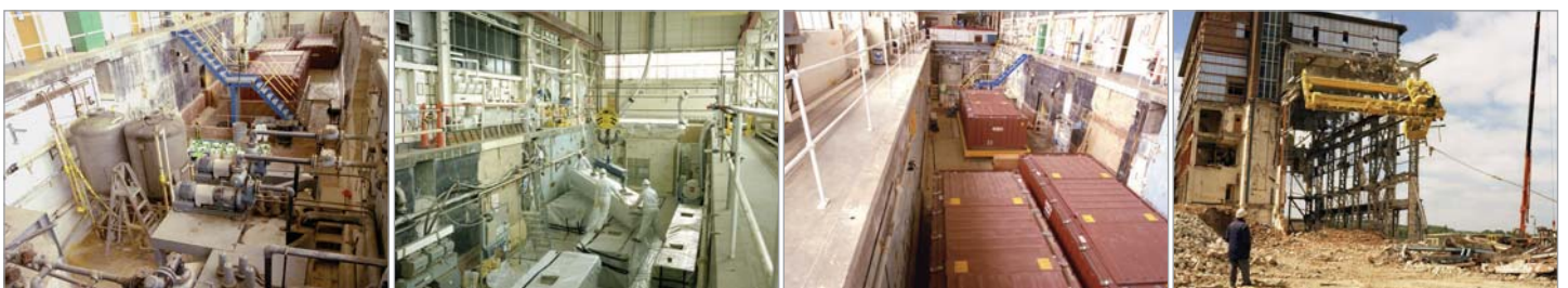
Before Dismantling Containers of LLW for the LLWR Facility demolition
