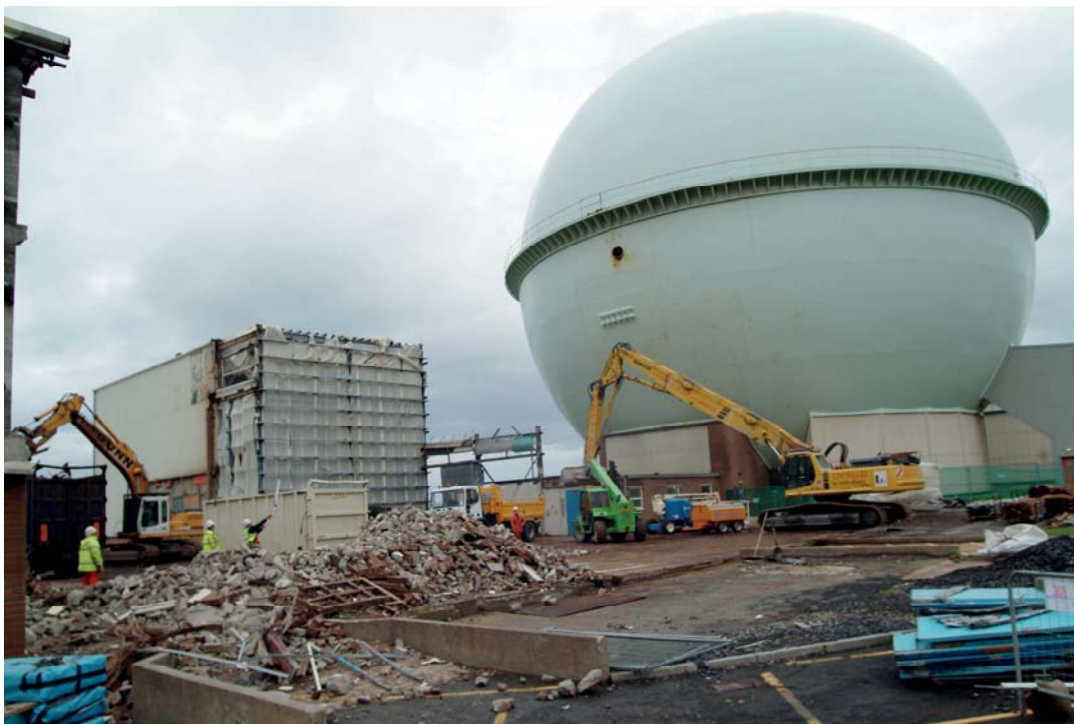
Figure 6.1: Decommissioning of DFR ancillary buildings
