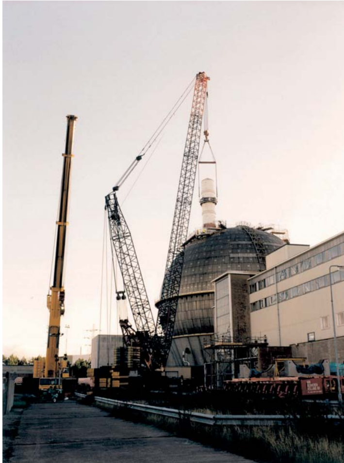
Figure 6.5: Decommissioning of WAGR
