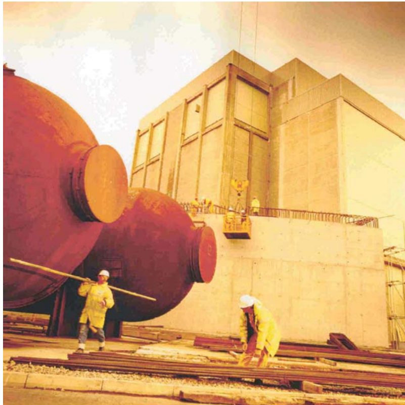
Figure 4.8 Decommissioning at Berkeley
