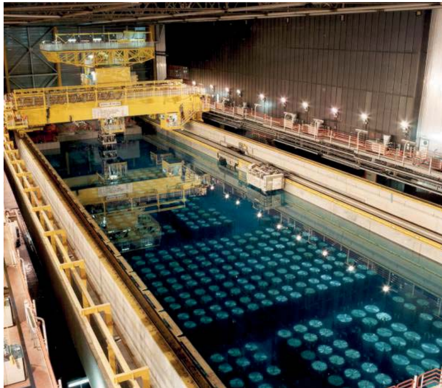
Figure 5.4: Oxide fuel storage pond holding multi-element bottles (MEBs)
