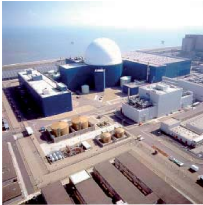
Figure 4.6: Sizewell B power station
