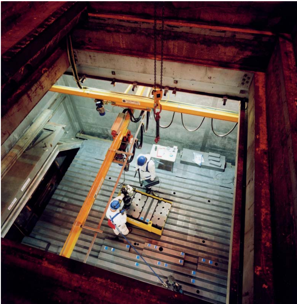
Figure 6.3: Removing graphite blocks during the decommissioning of the GLEEP reactor
