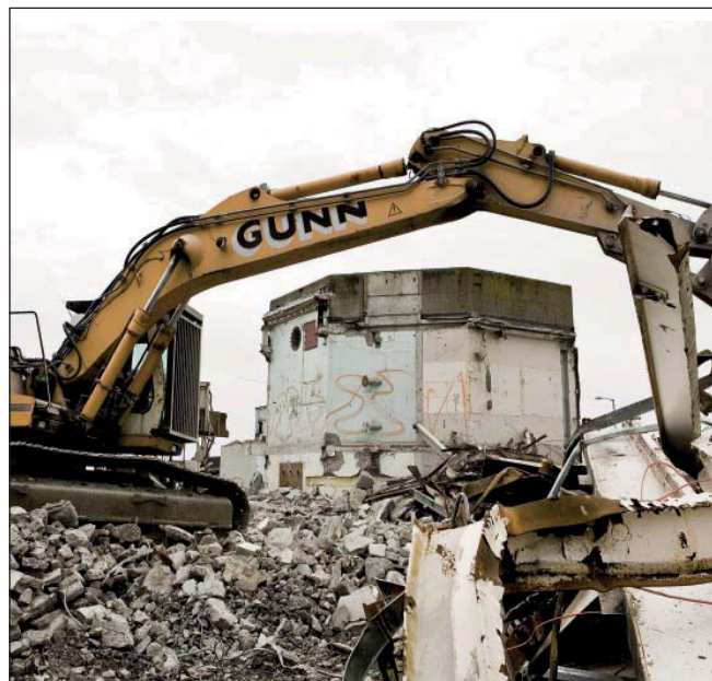
Demolition of nuclear facilities at Dounreay
