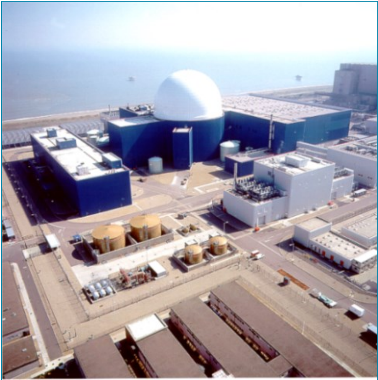
Aerial view of Sizewell B power station site
