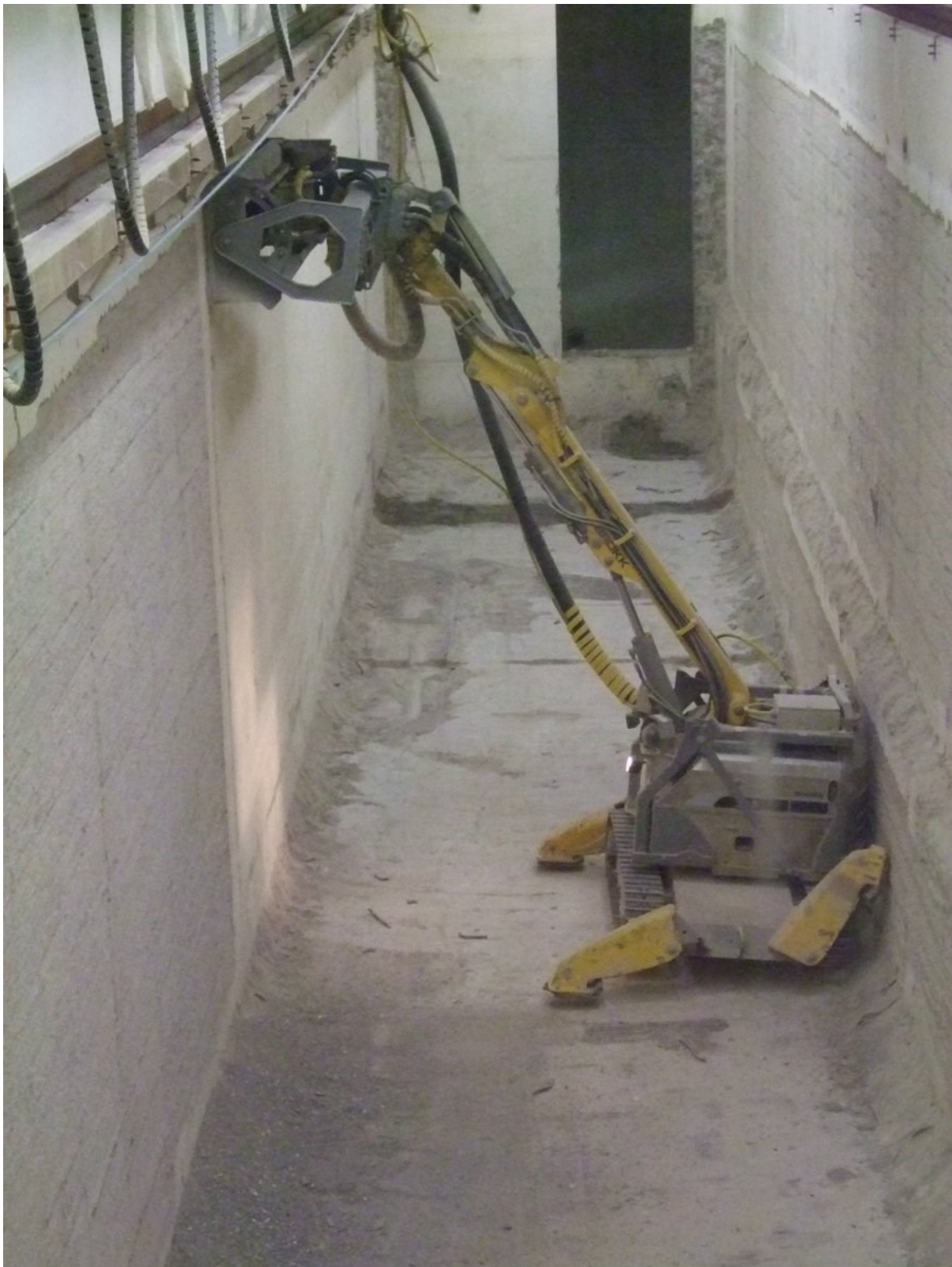
Robot removing surface-contaminated concrete
