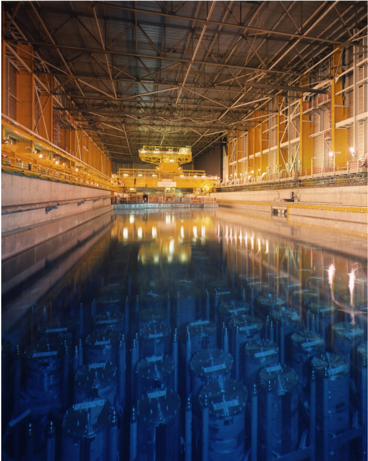
Spent fuel storage, Sellafield
