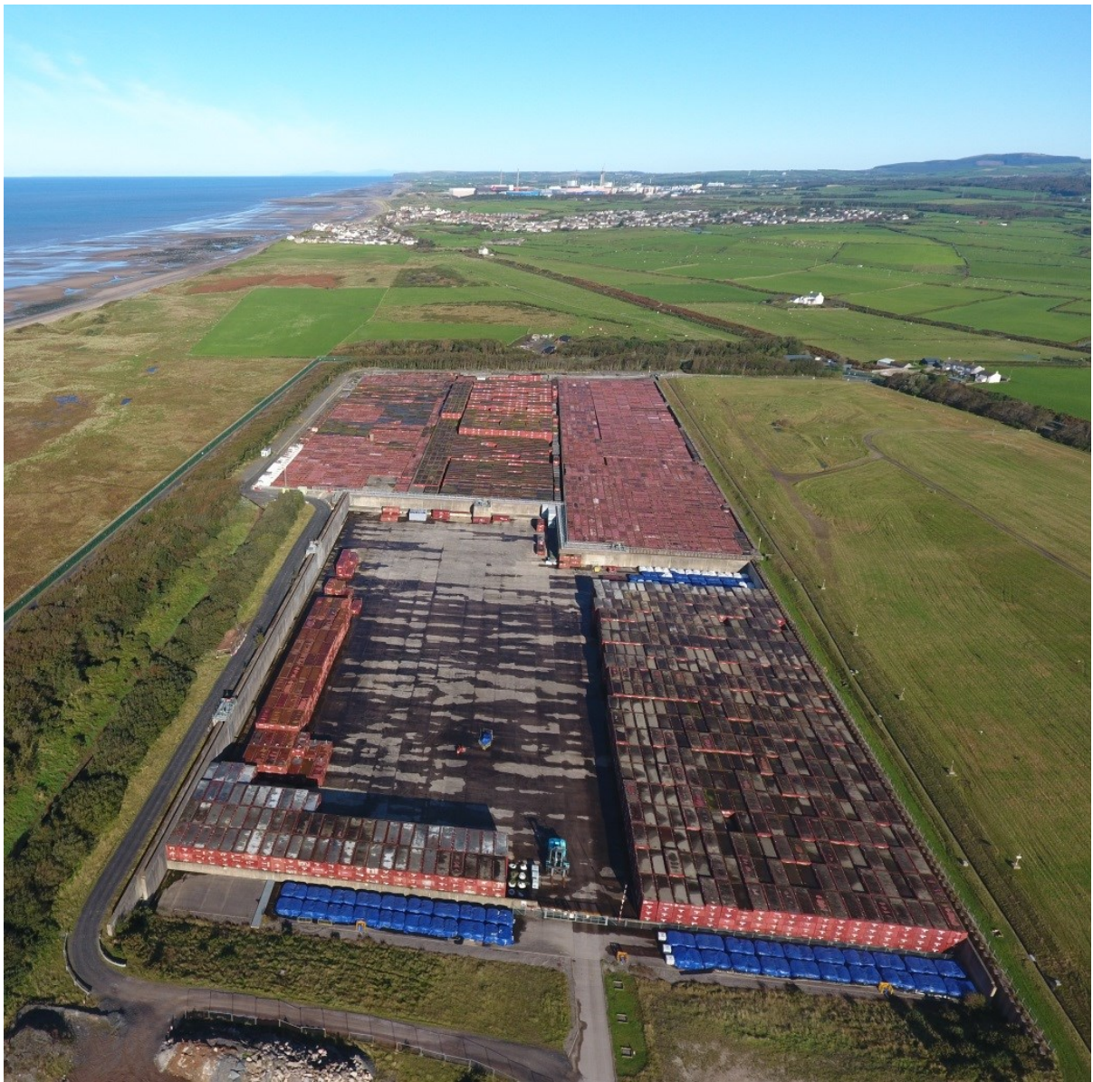
Aerial view of the Low Level Waste Repository, West Cumbria
