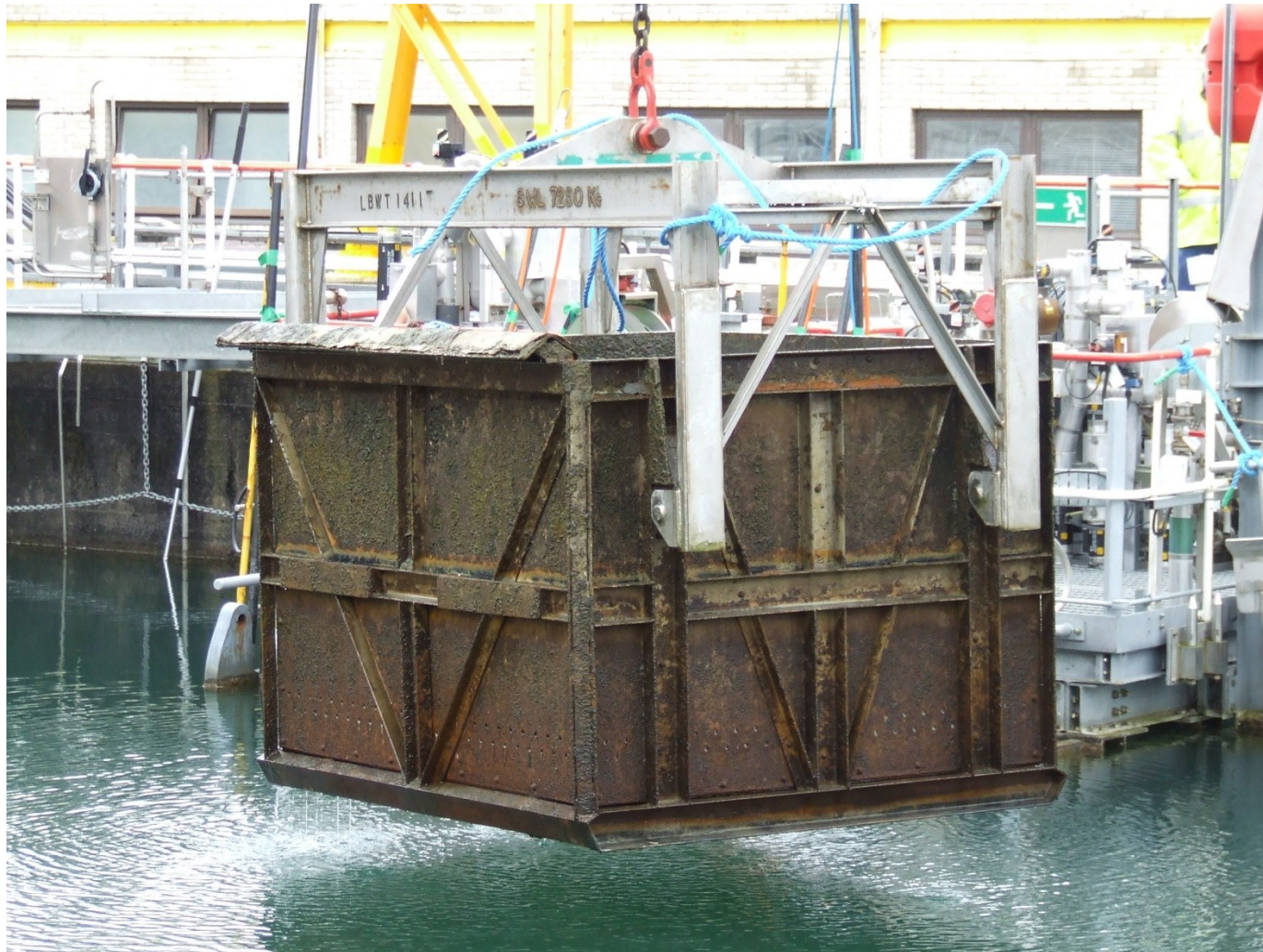
Fuel skip being removed from legacy pond, Sellafield
