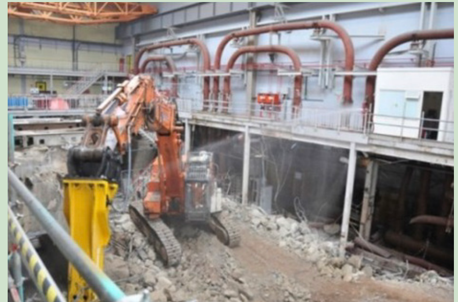
Image: Demolition work
