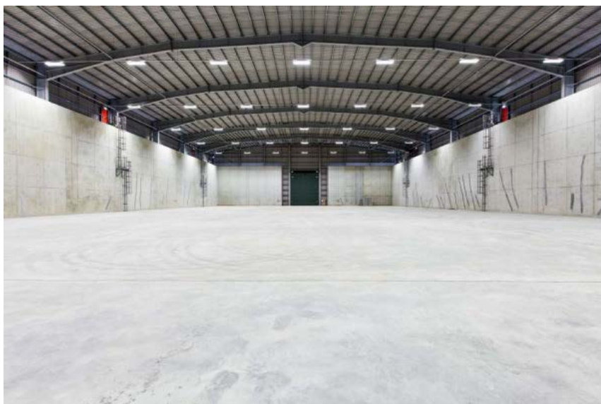
Internal view of empty Dounreay LLW disposal vault
