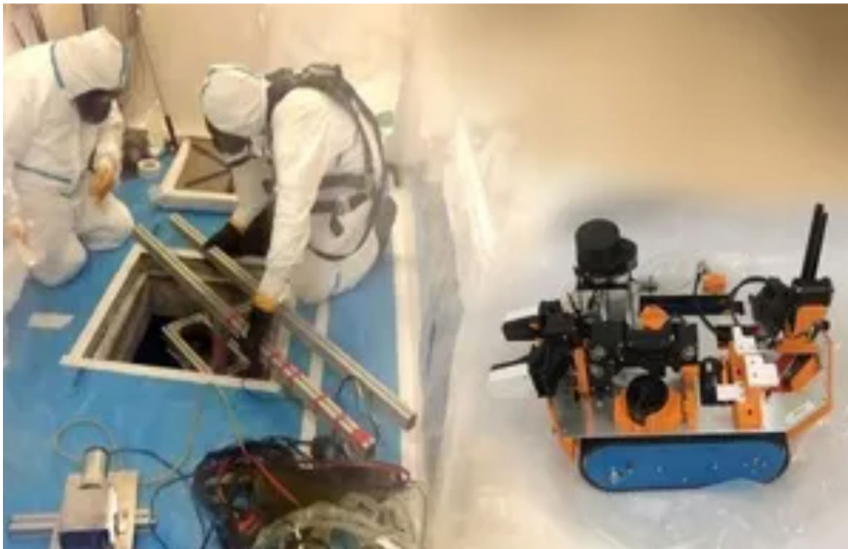
Robot assisting in decommissioning work
