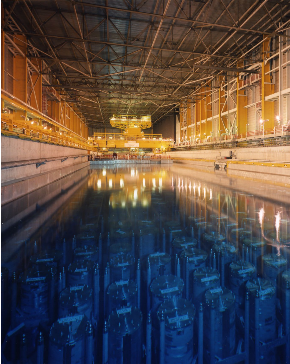
Spent fuel storage, Sellafield
