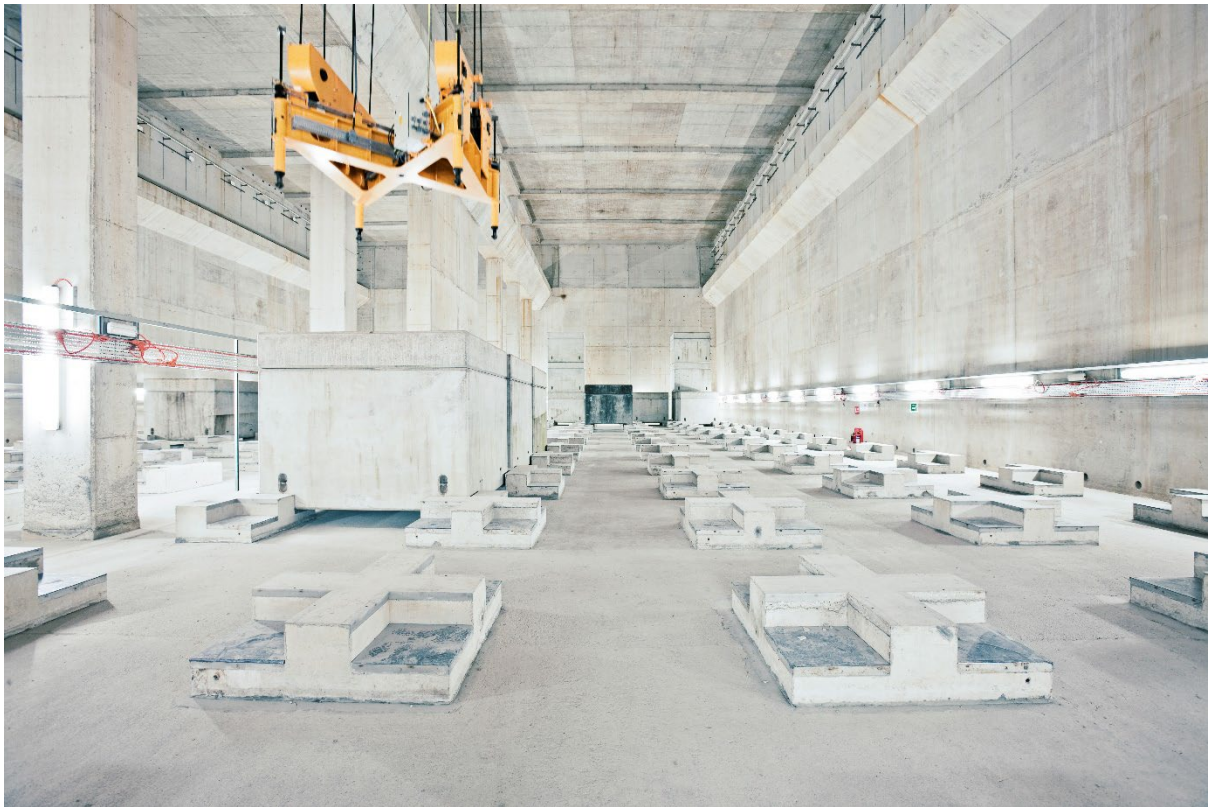
Inside the ILW store at Trawsfynydd
