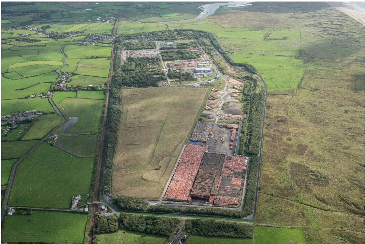
Aerial view of the Low Level Waste Repository, West Cumbria
